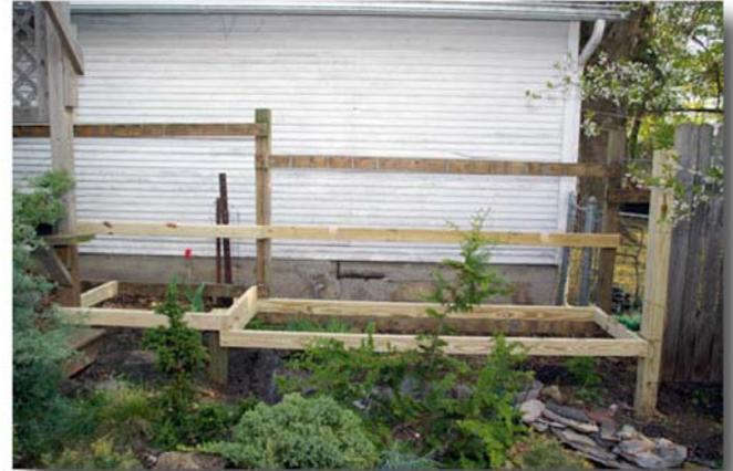
Construction involved first taking down the old fence section that was in need of removal and then building the framework strong enough to hold the weight of potted trees.
