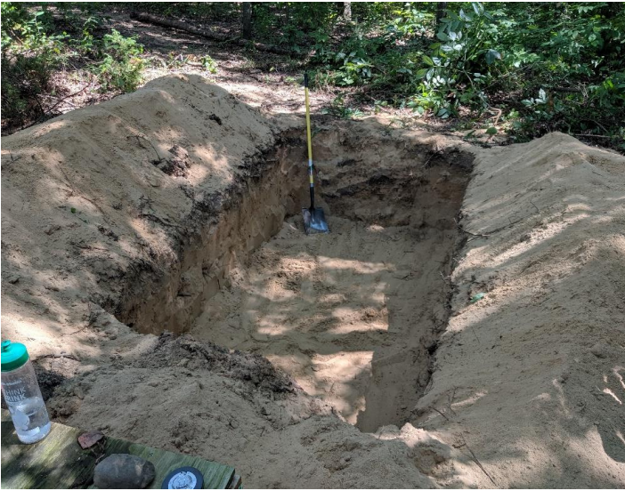
Big hole, oversized so I could assemble the walls in the hole.
