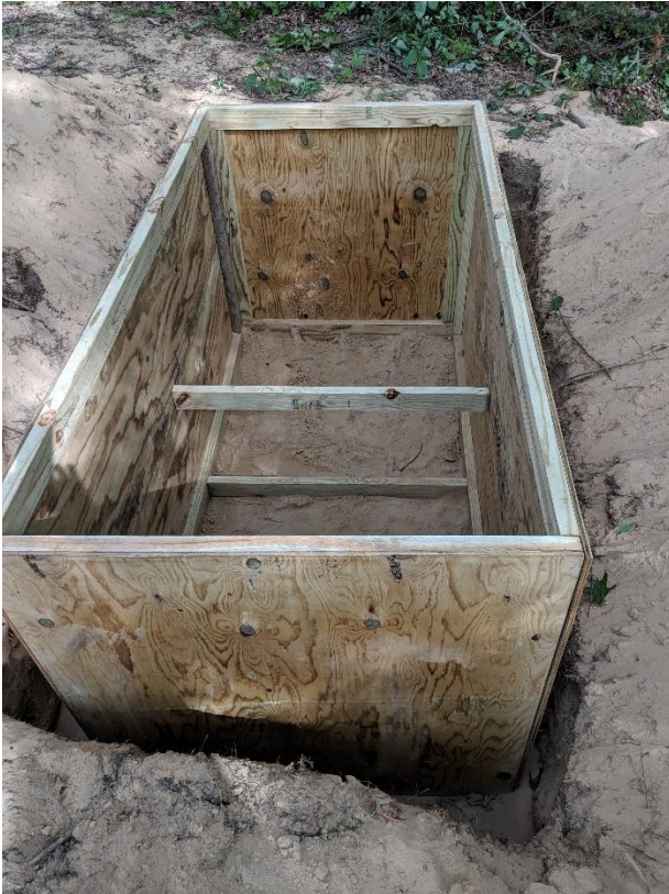
Walls are in and I add a brace 2x4 to keep the weight of the fill dirt from pushing in the sides. You will never keep the top square enough for the lids if you don't.
